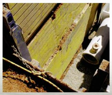
Vertical sheeting and trench support system for large OD pipe, box culverts and structures
